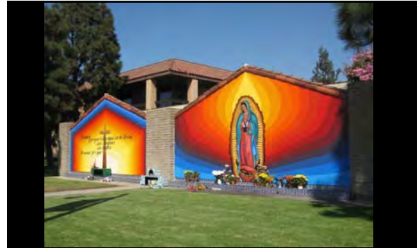
Housing Authority Office, Los Angeles Our Lady of Guadalupe , David Lopez, 1973 First Supervisorial District
